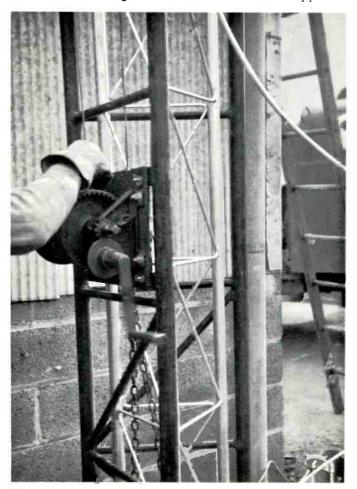
Kwik-Up Erector winch and unit with tower mounted inside. Section of tower mounted at this stage is ready to be hoisted ten feet to top of Erector.
