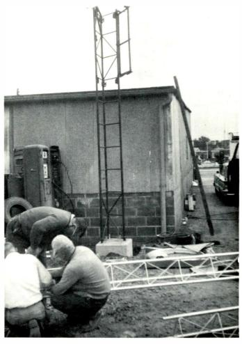
Kwik-Up Erector Kit installed on tower base and guyed, ready for first 30 feet of tower to be slid inside frame.
