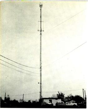
The 150 foot communications tower serves to repeat through 'channel B' the control center radio system over the entire county, and also serves to push the VHF-UHF systems operating for different county and civil groups over the entire county region.
