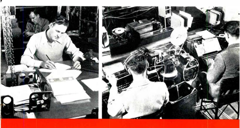
BEFORE RCA INAUGURATED ITS MODERNIZATION PROCRAM, THIS MANUAL METHOD OF CHECK-ING MESSAGES DESTINED FOR DELIVERY IN THE UNITED STATES WAS COMMONPLACE. OPERATOR AT LEFT TRANSCRIBES MESSAGE RE-CEIVED ON MORSE INK RECORDER TAPE WHILE THE ONE AT RIGHT PREPARES A MESSAGE FOR TRANSMISSION IN THE SAME MANNER.
