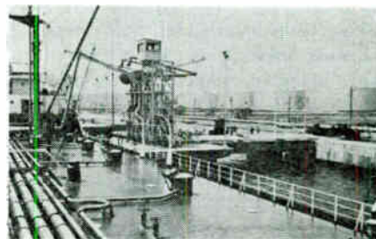
Discharging of crude oil from a tanker
