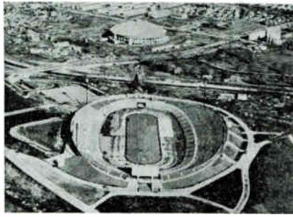
Makomanai speed skating rink (foreground) and indoor skating rink (background)
