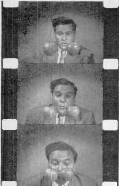
Scene from "How an Airplane Flies" —one of science films being made for color TV—shows how air blown between apples creates low-pressure area that sucks apples together. Color in such shows heightens interest, lets you actually see chemical changes, wildlife beauty.
