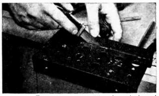
To save space, a strip 15" wide was backstwed from the standard 12" by 45" by 8" chassis. This was done after layout, drilling, and punching.
