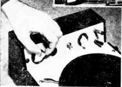
tube's filament. The entire chassis is mounted on a 6" by 6" steel sheet which is bent to fit below and in front of the control panel. To mount the chassis to the panel, bolt the toggle switch through both pieces, as shown in the drawing on page 153. Follow the same procedure with the antenna and ground jacks.
