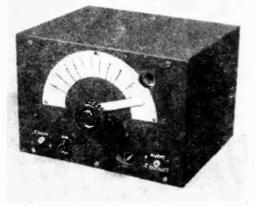
Housed in a trim cabinet, the original receiver had an extra input enabling it to be used with an FM tuner. A tuning eye is located beside the dial
