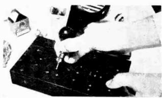
Punch and drill all holes before assembly. An electric vibrating tool easily marks a crackle finish, and lets you identify the sockets.
