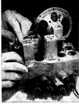
**Tubes are fragile, so install them only after** all the wiring is completed. The jumper lead from the RF section of C2 must be clipped to the grid cap of the 12A8 mixer tube.
