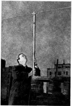
For best results the half-wave dipole should extend as high as possible above the building. A simple dipole and coaxial-cable transmission line is shown in Fig. 1. You can use other types of low-loss feeders in place of coax. Dipoles are directional; they favor signals coming from the direction of blocked arrows. operation and bring in difficult stations.
