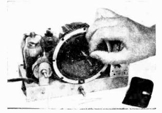
Three poper shims are inserted to center a loudspeaker cone
