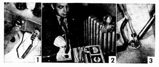
Before attempting to eliminate background hum from the record player, be sure that the trouble doesn't originate in the radio amplifier. A 100,000ohm resistance will simulate the pickup impedance. Good grounding is important to humless reception. If an ohmmeter test of the pickup case shows an imperfect ground, solder one end of a piece of wire to the holding nut, the other to the cable shield.
