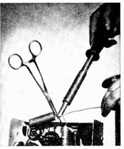
TEMPERED steel forceps that can be made to lock in one of several positions are particularly useful for holding wires or small parts in place while both hands are used for soldering. Slightly damaged or worn hemostatic forceps of the type illustrated above are available at many secondhand stores. Metal shims may be soldered to the blades to allow the right pressure for frequently repeated operations.—H. LEEPER.
