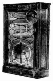
Above, the smallest packaged system: National Synfonette; right, the biggest: Electro-Voice Patrician. Former has little Danish all-range speaker, clever box, costs \$30. Latter has four speakers, including 18-inch woofer in Klipsch enclosure, two-level controls, four-way crossover, costs \$713
