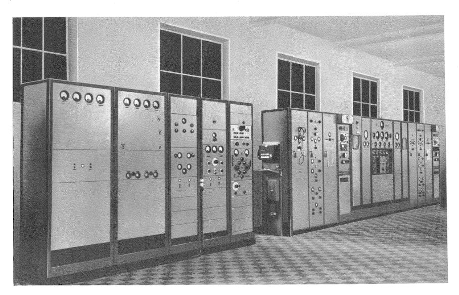
The single-sideband high-frequency transmitter in the illustration provides two telephone channels for the New York-Paris link and is installed at Pontoise, France. At the left is a 1-kilowatt driver and at the right is the 60-kilowatt output stage. The construction of this equipment by Laboratoire Central de Télécommunications is a logical result of its many years of work in this field.
