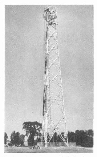
Fig. 17-200-foot wooden tower at Nutley, New Jersey.
