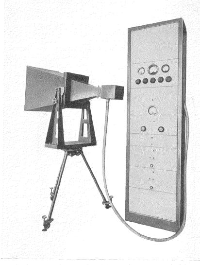
Fig. 12-9-centimeter receiver of the Paris-Montmorency radio link.
