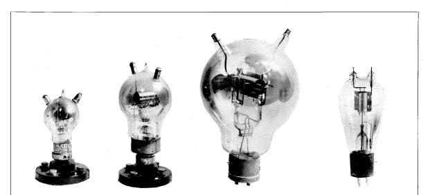
Fig. 12—Special Valves for High Frequencies—Left to Right : French 10 Watts and 50 Watts, 1920; Tungsram Type O, 200/2 500, 200 Watts, 1937; Standard Telephones and Cables Type 4304-B.
