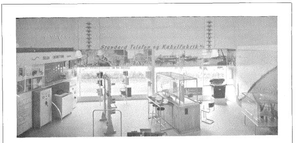
THE STANDARD TELEFON OG KABELFABRIK A/S AT THE OSLO EXHIBITION, 1938 The stand included a model of the 7.A2 Rotary System equipped with Automatic Ticketing facilities enabling a call to be made from the exhibition to any Oslo subscriber and producing a ticket giving complete data of the connection.
