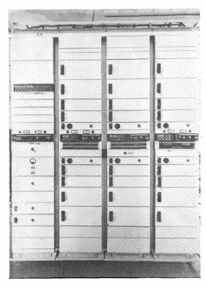
Fig. 13—Bay Containing Equipment for Six Carrier Channels.
