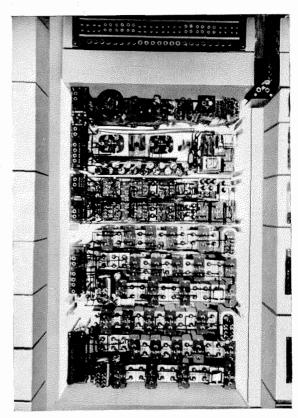
Fig. 2—Equipment for Single Channel Carrier Telephony.
