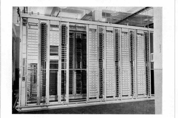
Fig. 5-Galati 7-D Exchange-1st Line Finders, Final Selectors and Penultimate Group Selectors.
