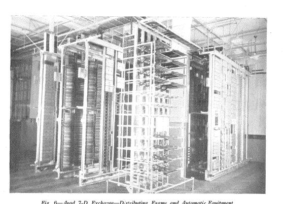
Fig. 6—Arad 7-D Exchange—Distributing Frame and Automatic Equipment.
