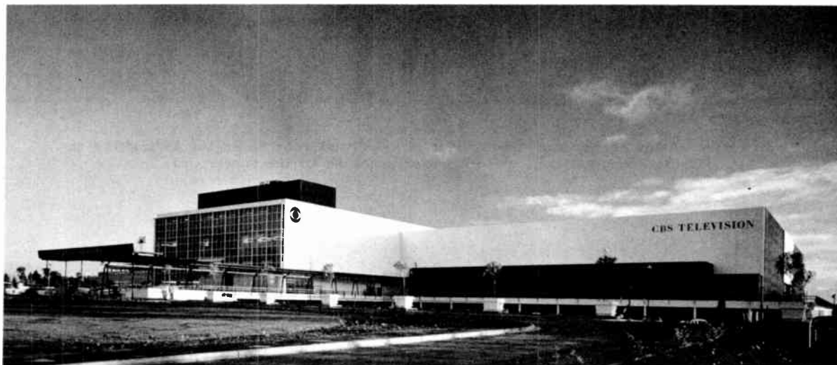
Fig. 1 CBS Television City - the studio building at the right houses four one-quarter acre studios; the three-story, glass-walled structure to the left is a service building housing scenery shops, maintenance facilities, and offices.
