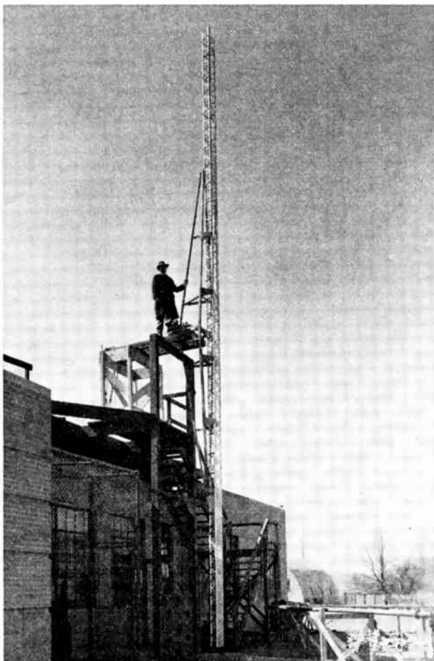
Fig. 7—A close-up of one of the uni-directional transmitting antennas
