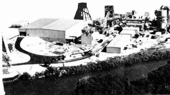
[3] By heating light-fraction refuse in an oxygen-deficient atmosphere, gas or oil can be produced (pyrolysis). The plant shown here, which was recently completed by Monsanto, features a rotary kiln in place of the vertical shaft furnace depicted in the diagram. Rated at 900 tonnes per day, the facility furnishes steam to Baltimore, Md., for electric generation.
