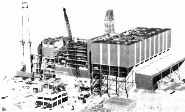
[1] No "prior processing" is required to burn waste in a typical moving-grate combustion boiler. The 1080-tonne-per-day Weelabrador-Frye refuse-energy plant shown here went on-line in September 1975, sending steam to General Electric's Lynn River (Mass.) Works. This is the first privately owned and operated refuse-energy plant in the U.S., and it will serve 16 North Boston communities.
