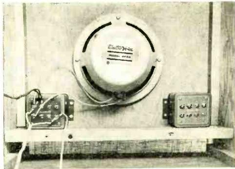
A peek inside of an unfinished bass reflex cabinet shows the two University N-2A crossovers attached to the front panel. See the wiring diagram above.
