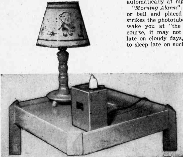
**The Light Switch** in use. The lamp is controlled by light passing through the window in the box.
