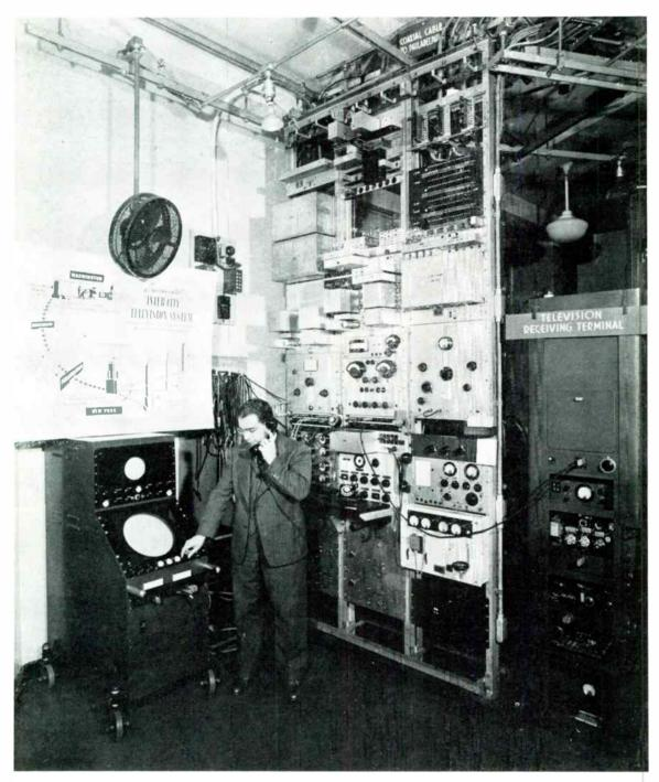
FIG. 10. NEW YORK CITY TERMINAL OF THE N. Y.-WASHINGTON COAXIAL CABLE. TELEVISION SIGNALS ARE MONITORED HERE, THEN CONDUCTED TO ANY OF THE TELEVISION BROADCASTING STATIONS IN THE CITY
