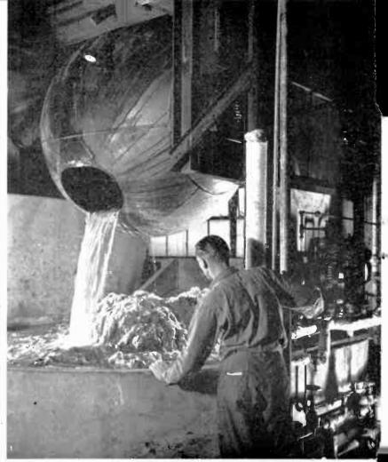
FIG. 3. THE HUGE BOILER ABOVE IS EMPTIED INTO THE WASHER BELOW, WHERE IMPURITIES ARE REMOVED
