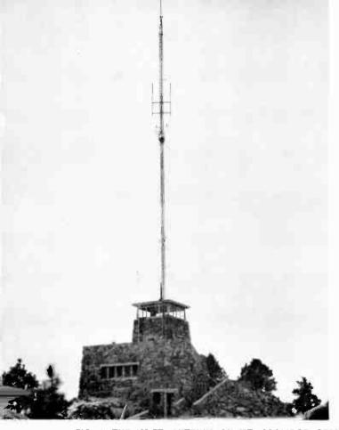
FIG. 4. THE 125-FT. ANTENNA ON MT. COOLIDGE. BEAM ARRAYS ARE FOR COMMUNICATION WITH RAPID CITY
