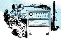
Coll Laboratories designed and Western Electric produced more than 1600 electronic gun directors and gun data computers which greatly increased the accuracy of anti-aircraft and coast defense guns.
