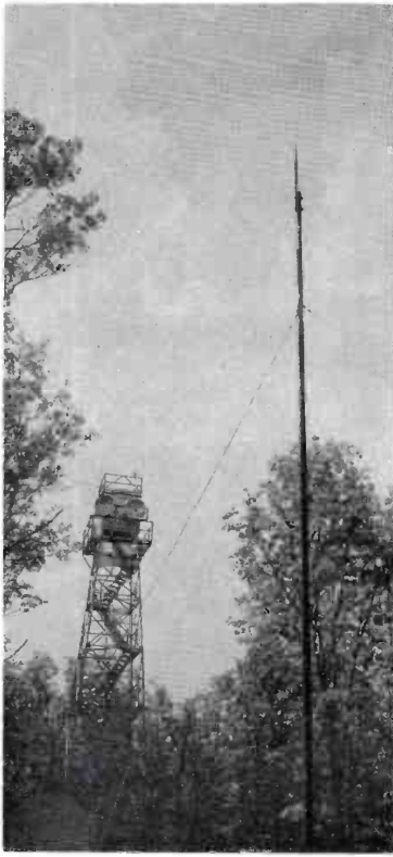
THE CONESTOGA RELAY STATION, WITH THE ASSOCIATED VHF ANTENNA IN THE FOREGROUND
