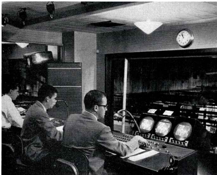
FIG. 11. PERFORATED ACOUSTIC BOARD, APPLIED OVER ACOUSTIC BLANKET ON CEILING AND WALLS OF CONTROL ROOM, AFFORDS ADEQUATE SOUND TREATMENT AND IS PLEASING TO THE EYE AS WELL
