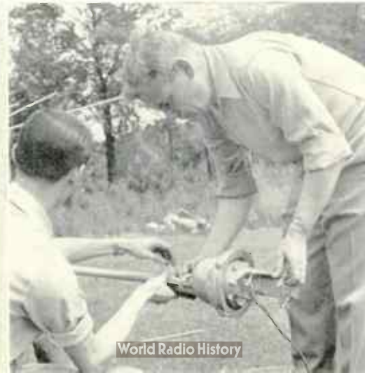
Fig. 10. Clamping rotator to pipe.
