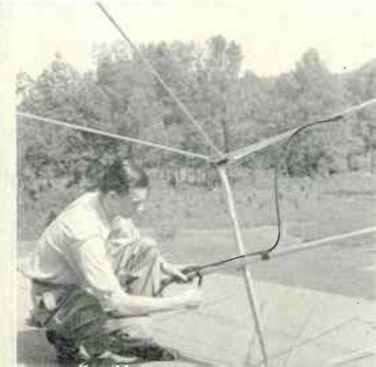
Fig. 11. Taping line prevents strain on connection
