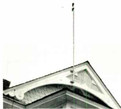
Fig. 2. Stacked vee is simple, efficient
