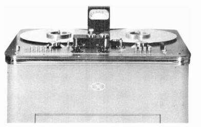
Fig. 1. Top deck of the studio recorder, ready to take the tape reels
