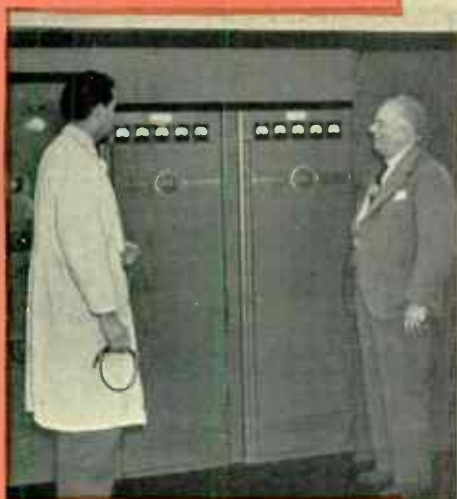
TWO FEDERAL 250-WATT TRANSMITTERS assure 24-hour service. One is in continuous service—the other stands by in case of emergency. Sgt. J. A. Stoltenberg, Police Radio Engineer (left) and Police Commissioner Hamilton R. Atkinson.
