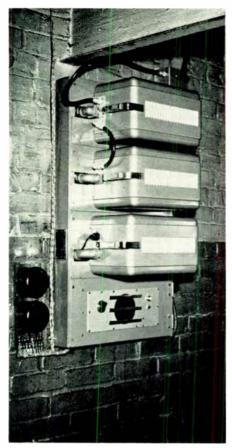
FIG. 8. INDUCTION RECEIVER AND TRANS-MITTER AT MICHIGAN CENTRAL TOWER
