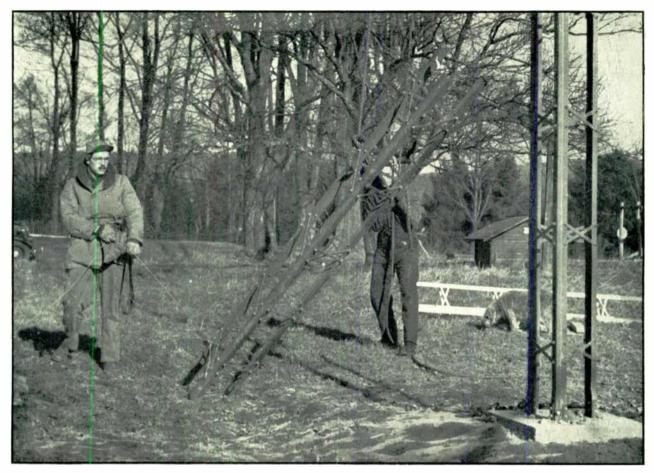
FIG. 1. HOISTING ROPE IS ATTACHED JUST ABOVE MIDDLE OF MAST SECTION. SMALL LINE STEADIES SECTION ON WAY UP
