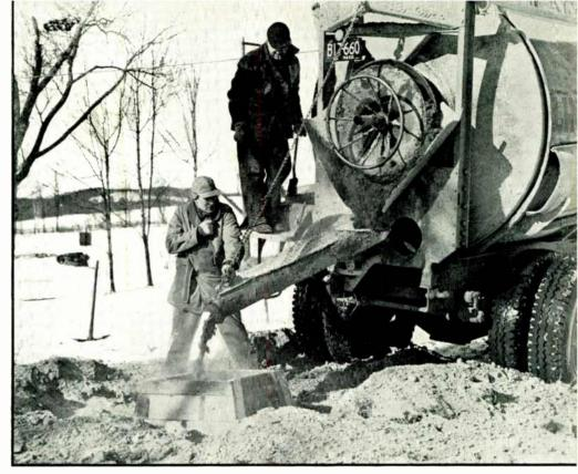
FIG. 7. POURING CONCRETE INTO THE FORM FOR THE BASE OF THE TOWER
