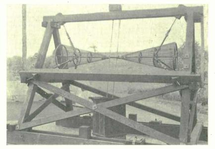
FIG. 32. CONICAL DOUBLET USED AS THE PICTURE TRANSMITTING ANTENNA
