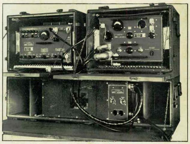
THE LINK 250-WATT FM CARRIER TRANSMITTER USED FOR MILITARY RELAY COMMUNICATION NETWORKS
