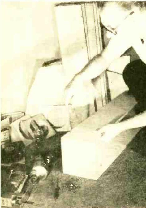
**FITTING** the four 33x7½x½-in. plywood sides together with screws is the first step.
