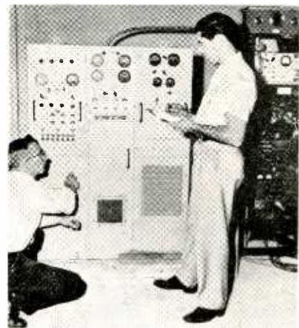
Operator at left is adjusting power supply of amplifier-modulator while co-worker records data. Left to right are the power controls, r-f amplifier and radio modulator. Transmitter is at the right
