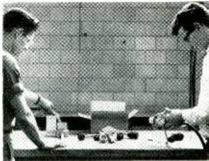
**STEP 3**—Wired connectors are dipped in solvent-type cleaner as at left, then dried with filtered air at right. Jet spray is now used instead of dip here
