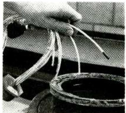
**STEP 9—Sealing pigtail by dipping in hot plasticized ethyl cellulose**
