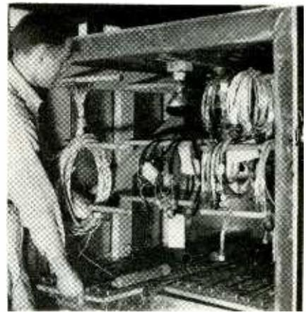
**STEP 8—Heat lamps provide 120 F temperature for 2-hour cure cycle in oven**
