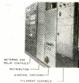
application and removal of power, gradual increase of filament voltage, sequencing of d-c voltages, voltage and temperature monitors, indications and alarms for quick trouble shooting, detection of power line transients, and automatic or manual marginal checking for the detection of weak components. Check 408 on Reader Service Card.
