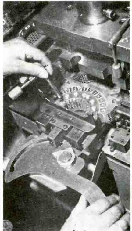
STEP 2—With bank assembly in position on slide, operator inserts positioning pin. Right hand is on lever which will later be pulled to move slide under press
