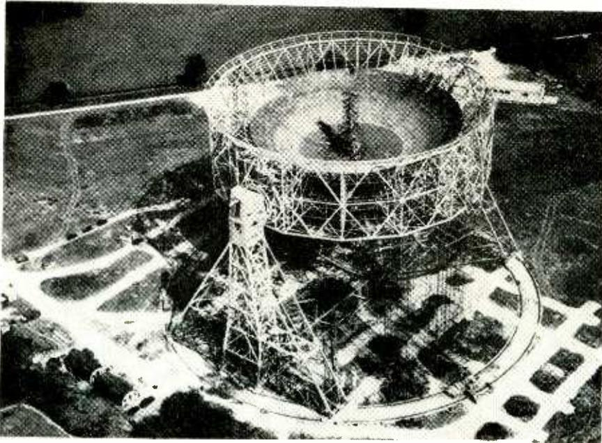
**ANTENNA**, mounted on tower in center of a reflecting surface cradled in a 250-ft diameter bowl, will pick up sources of radio emission 200 million light years ago when latest development in . . .
