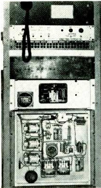
New automatic changeover controls are in lower half of rack, with modified remote control unit at top. Carrier loss for 8 seconds initiates shift
