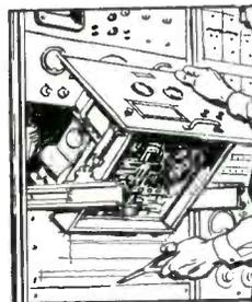
*Five seconds to put chassis in testing position. Slides smoothly out of rack, locks. Pivoting mechanism brings under-chassis parts to easiest working angle. Functioning of unit need not be interrupted!*
