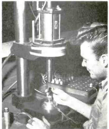
Placing guide thimble over stator in fixture on air-actuated arbor press
