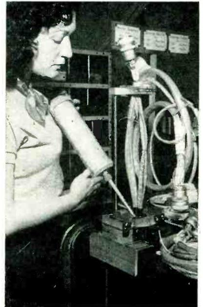
Filling steel radar assembly mold for large connector in Baltimore plant of The Glenn L. Martin Co.
