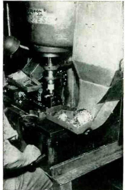
Sheet-metal hoppers alongside press feed brass shafts and supports, for riveting together when loaded into press manually. Note semicircle cut into bolster, with chute below leading to tote box for finished pieces. Spring clips welded to hopper at right can be used to hold work cards
