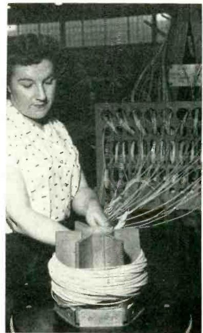
Air motor under bench turns arbor slowly to wind wires for cable as they are pulled off pegs of storage rack in background through holes in vertical plywood board. When winding is completed, operator pulls taped end of cable out from behind paddle board and lifts off the coiled cable
