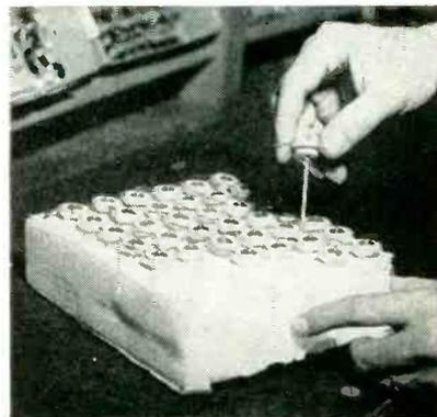
Removing special capacitor from foam plastic shipping block
