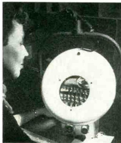
Magnification combined with intense illumination improves efficiency of inspecting screw terminals in missile black box
