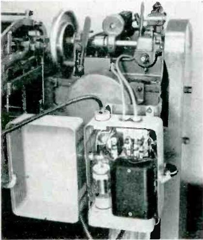
**SLOW, CUSHIONED AUTOMATIC START** Electronic speed-control automatically and smoothly accelerates the winding arbor to required speed and maintains it. No "jockeying" needed by operator. Wire breakage is minimized, tension is uniform.
