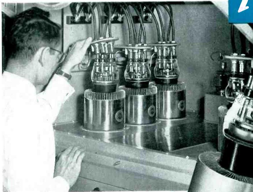
Installation of Federal F-8C25 power triodes in modulator tube compartment of 207B-1 transmitter.
