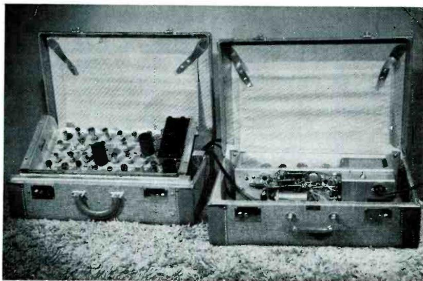
Complete rack-panel equipment in carrying case (left) with associated regulated power supply operating from 117-v outlet (at right)
