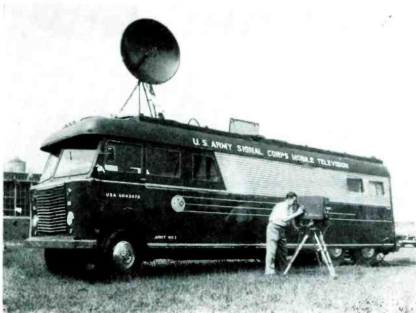
Complete transmitting studio for the Signal Corps is equipped with a specially constructed operating desk for the portable monitoring, control and power supply units used with the field tv cameras
