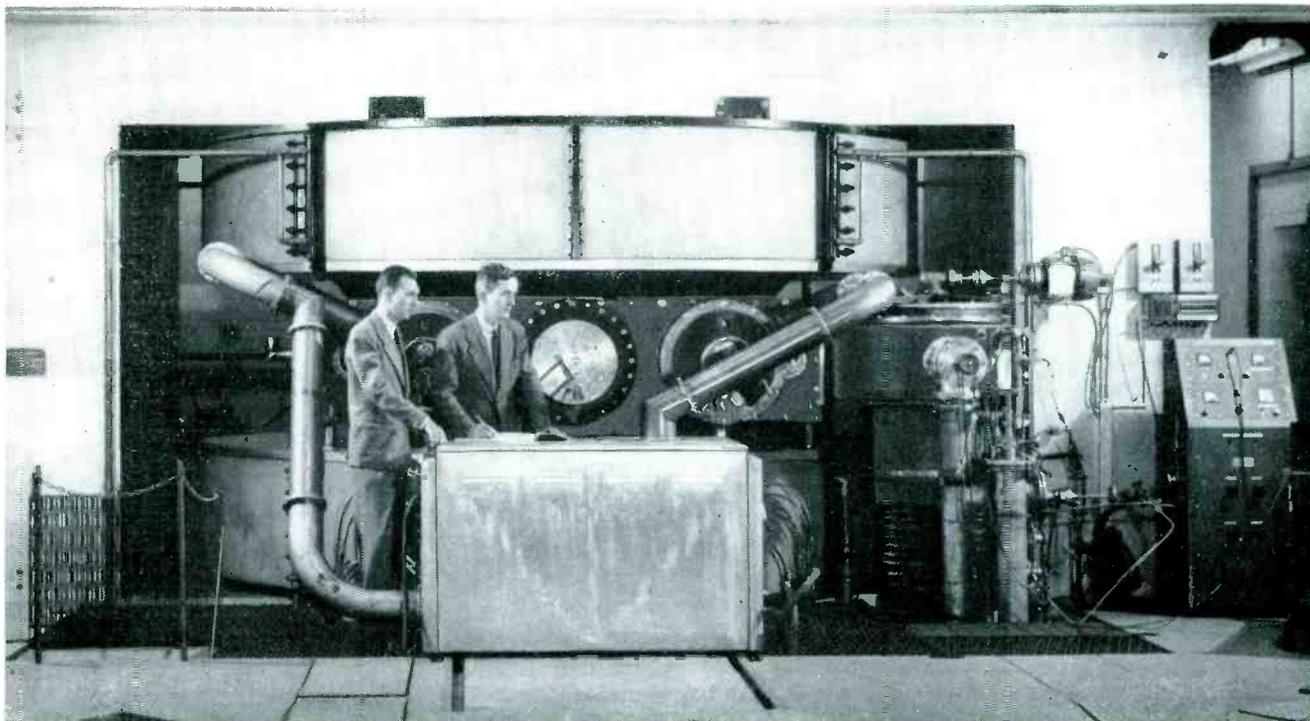
Complete r-f setup with dee in place between magnet poles. Cathode line at right and plate at left
