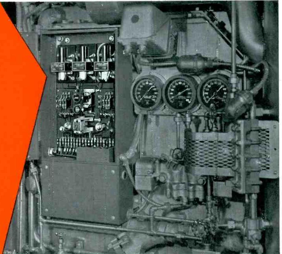
The three ADLAKE Relays in this steam generator control, manufactured by The Adams & Westlake Co. for Combustion Engineering-Superheater, Inc., were designed for foolproof operation. For, in addition to their timing, load and control functions, they have an important safety job to do (see panel).
