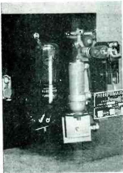
Vacuum-tube relay unit. Phantom view of cover was obtained by taking two exposures on same negative, one with and one without cover
