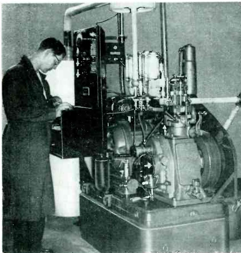
Knock-testing engine in Ethyl Corporation plant, using Malraison Mixture Thermostat for maintaining temperature of gas-air input mixture within 2 degrees of  $300^{\circ}\text{F}$  as indicated by mercury thermometer. Vacuum-tube relay housing is mounted behind control panel at eye level
