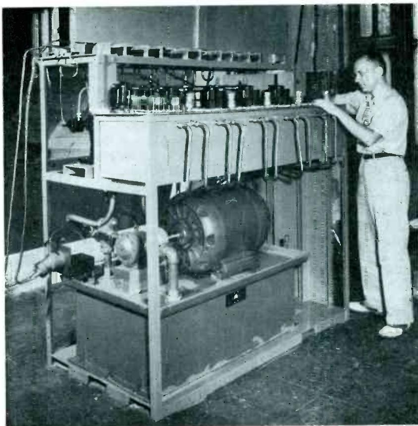
Complete setup of electronic and hydraulic units that connect to the printing press. Five 24-tube chassis are being immersed in oil inside the long steel box in which they normally operate
