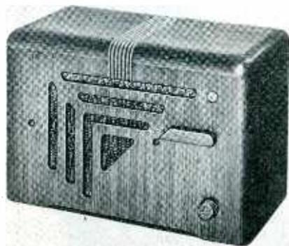
cabinet with volume control and indicating pilot light. Up to sixty stations can be operated together as a system. Operates from either a.c. or d.c. lines of 110 volts.
