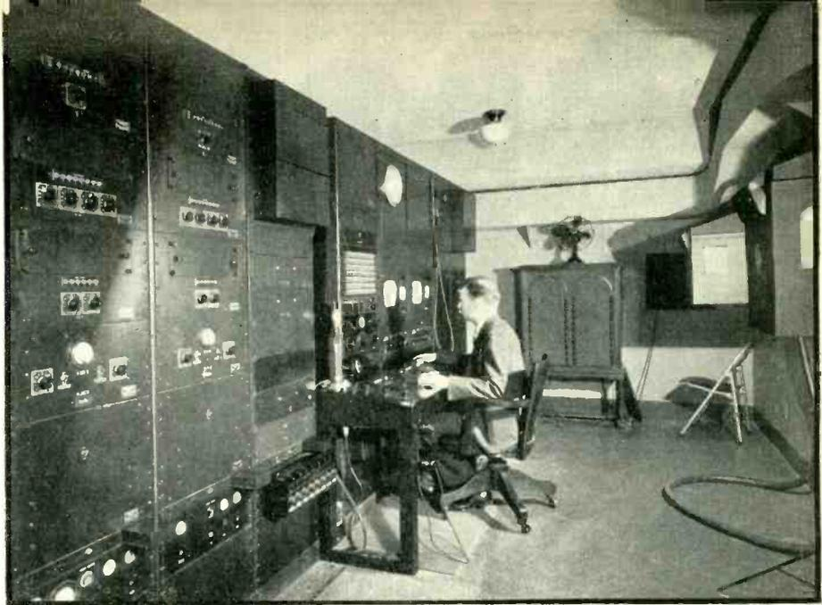
The film-projection room is fitted with monitoring apparatus for two video and audio channels, one for each projector, so that continuous film programs can be handled.
