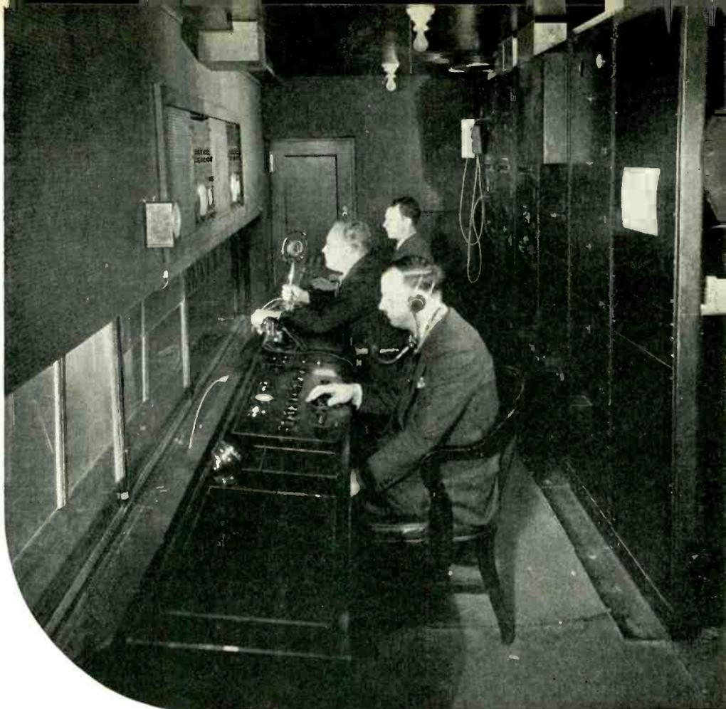
◀ The control booth contains three positions, for video, general production and audio monitoring, arranged before a window overlooking the studio below. Note the "Kinescope" monitors in front of the video and production operators
