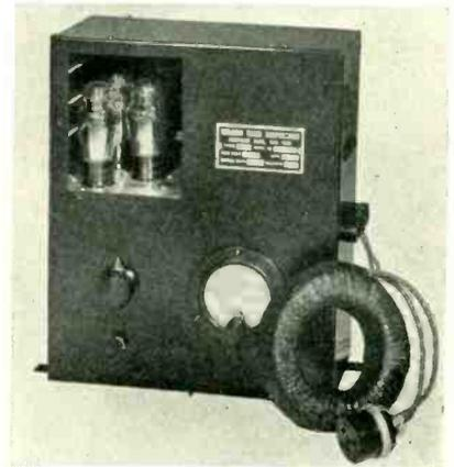
meter shunted across the condenser to determine the condenser charge. The instrument has three ranges, obtained by shunting the transformer secondary by resistors of different values. The instrument is calibrated in r.m.s. values of current. In operation the primary lead to the electric welder is passed through the doughnut shaped coil which forms the current transformer.
