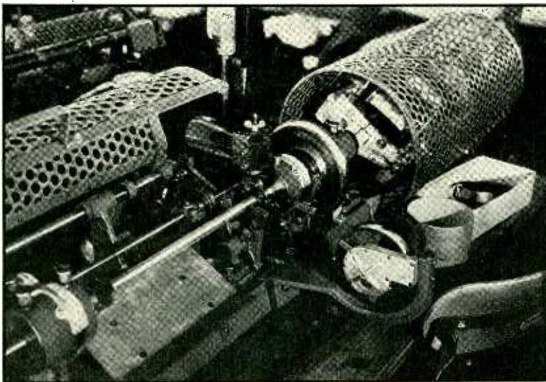
A grid winding machine at the Radiotron plant at Harrison, N. J. The English practice is identical in its essentials to that shown above
