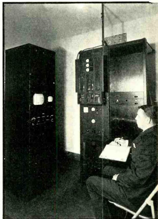
*The radio relay transmitter at the RCA Building which transmits the video signal on 177 Mc. to the main transmitter in the Empire State Building*
