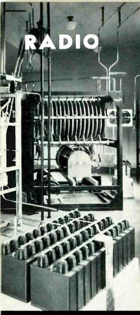
*Final amplifier tuning equipment and transmission line at KOA, the 50 kw. NBC station at Denver*
