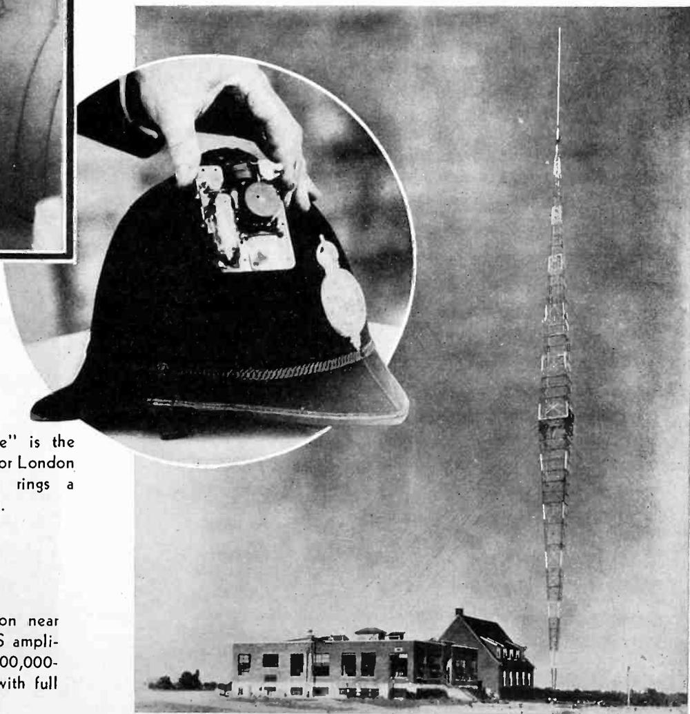
A tiny Marconi "valve" is the feature of this head-set for London policemen. A relay rings a bell for calling.
