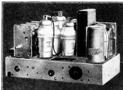
Chassis of **AUDIOLA AUTO RADIO** in which tubes are shielded with Goat form-fitting Tube Shields.
