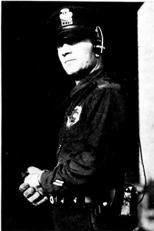
A miniature radio receiving set invented by Ralph O. Gordon of Los Angeles, to be worn by policemen on their beat. The set is worn on a Sam Browne belt with an earphone attached to the cap, the whole weighing less than three pounds.
