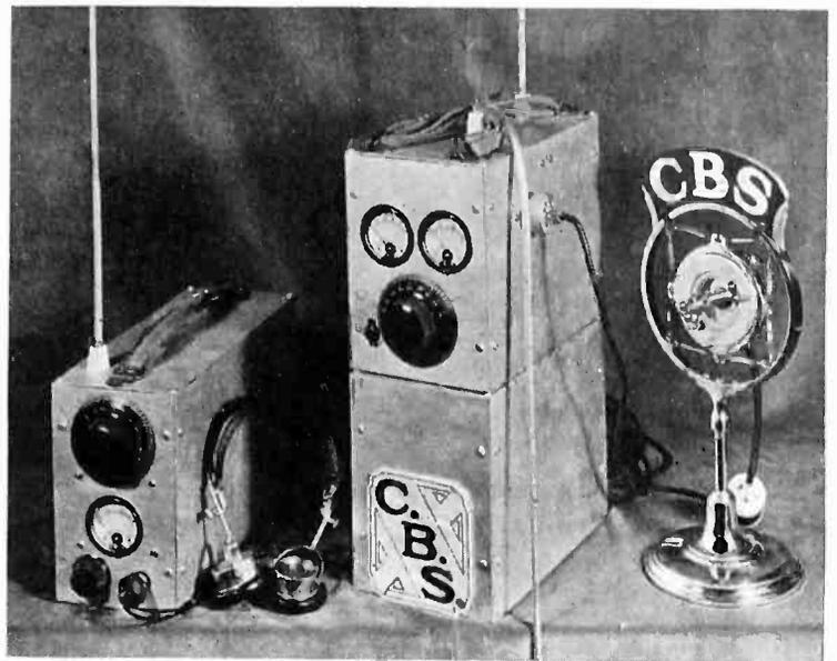
Ultra high-frequency portable transmitter and receiver, working on 40-60 megacycles
