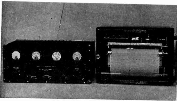
Automatic field-intensity recorder used for continuously monitoring WJSV
