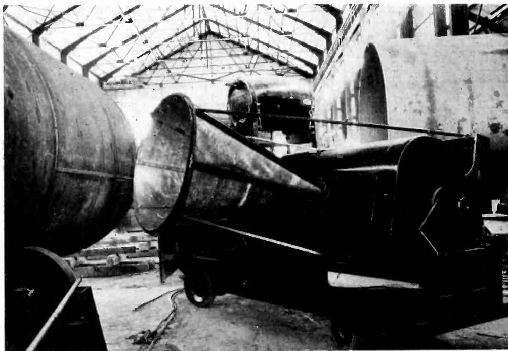
X-raying the  $2\frac{3}{4}$ -in. plates of the Boulder Dam steel conduits for faulty welds
