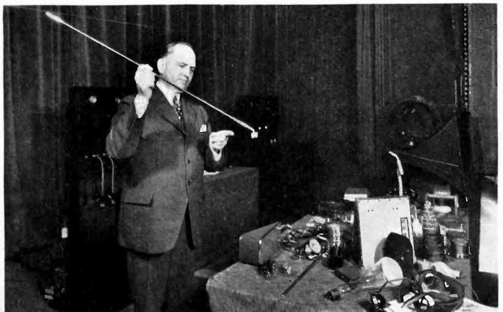
Sergius P. Grace, of the Bell Telephone Laboratories, is holding a permalloy rod in a north-south direction. In this position, due to the earth's magnetic field, the rod becomes a magnet of sufficient power to hold up a block of steel which falls when the rod is moved from its position
