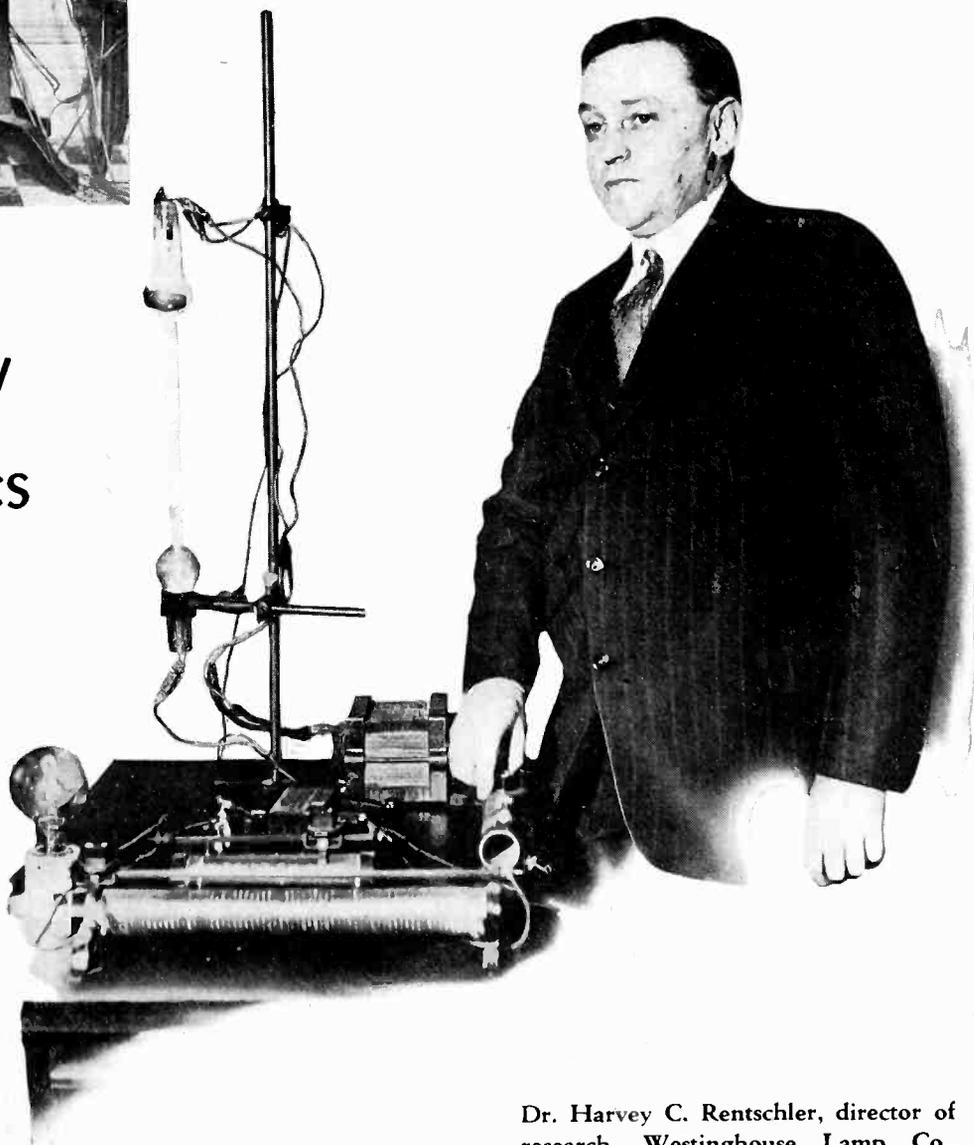
Dr. Harvey C. Rentschler, director of research, Westinghouse Lamp Co., demonstrates new sodium-vapor tube lamp which is three times as efficient as neon tube. Formerly sodium-vapor tubes quickly blackened and became useless; invention of new glass by Dr. Pirani, Berlin, avoids discoloring
