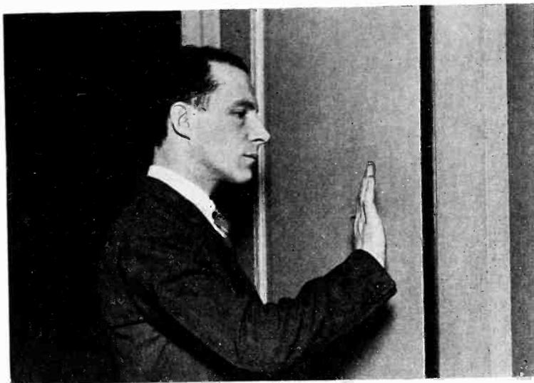
Professor Theremin now opens doors, starts machinery, with a wave of his hand. Door shown will follow his body at 2-inches distance. If he stops, it stops. Only the plate shown is sensitive; wire leading to it is inert and can be handled bare without effect
