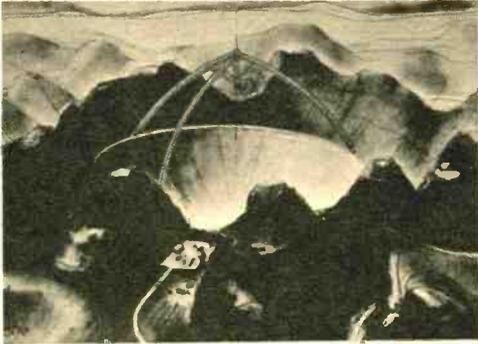
Below is working model of fabulous 1000-foot wide radar, designed by Cornell U. for construction in Puerto Rico (see artist's conception, left). It will explore cloud-covered Jupiter, more than 400-million miles away. Model was built by G. M. Zeitlin, shown holding driven element which is suspended above dish.
