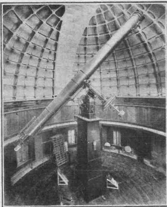
The 36-inch telescope of the Lick Observatory with which the observations were secured is shown in the above photograph.
