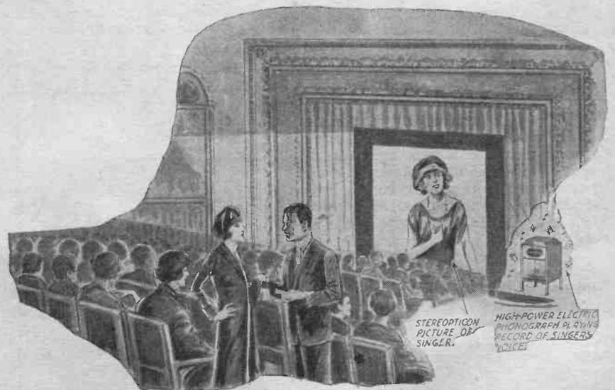
In the smaller theater a "talkie" substitute is used with good results. The system is illustrated above and employs a stereopticon picture of the singer and an electric phonograph employing a powerful amplifier, upon which a record of the singer's voice is played. While this method is not as realistic as legitimate talking pictures, it forms an excellent substitute.
