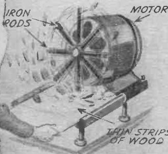
THE CRACKING UP OF AN AIRPLANE PORTRAYED BY BREAKING THIN STRIPS OF WOOD WITH MOTOR DRIVEN IRON RODS
