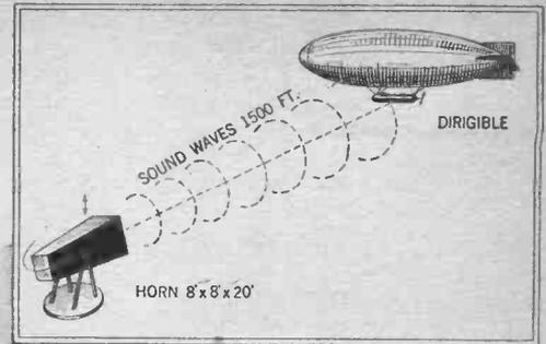
The above illustration shows the position of the large horn and dirigible during the experiment described here. The horn measured 8 ft. x 8 ft. x 20 ft. The dirigible flew above the horn at a height of 1,500 ft., and those on board distinctly heard voice as well as musical programs. The photograph at the left shows the huge horn mounted on the roof of the Victor Talking Machine Co. plant, at Camden, New Jersey.
