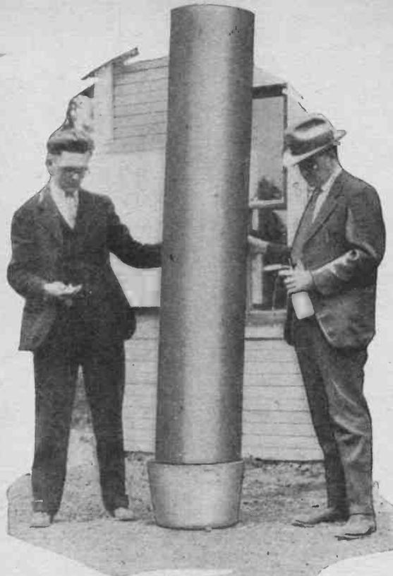
**T**HIS chamber is to be released through the torpedo tubes or through suitable hatches. It can be made of a very thin metal and an internal pressure is used to counteract the external crushing pressure. The chambers are to be nested, and each supplied with covers containing soda-lime.
