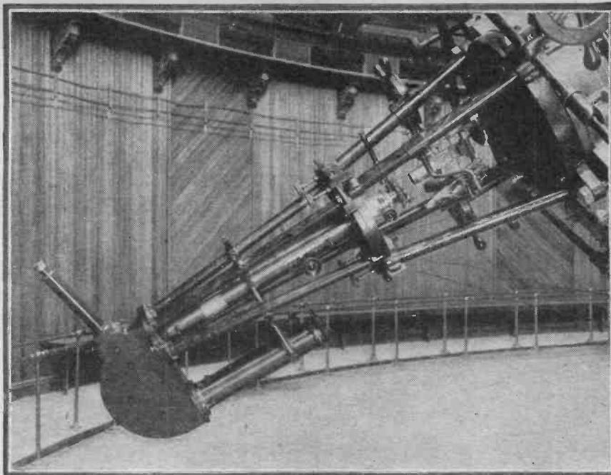
*The photograph at the left shows the "Mills" three-prism spectrograph attached to the 36-inch Lick refractor.*
