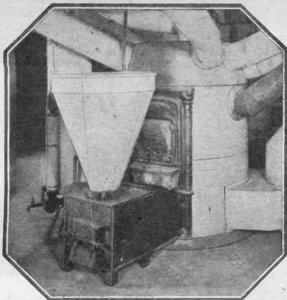
The photograph above shows a typical sawdust burner used for heating houses in Washington and Oregon. The sawdust hopper is the funnel-shaped arrangement attached to the front of the furnace. The small door at the bottom is the draft control. The heat is regulated by the amount of air admitted.
