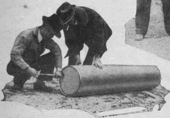
Pumping air into the can. The other end is also sealed. The side through which the man entered remains beneath the water.
