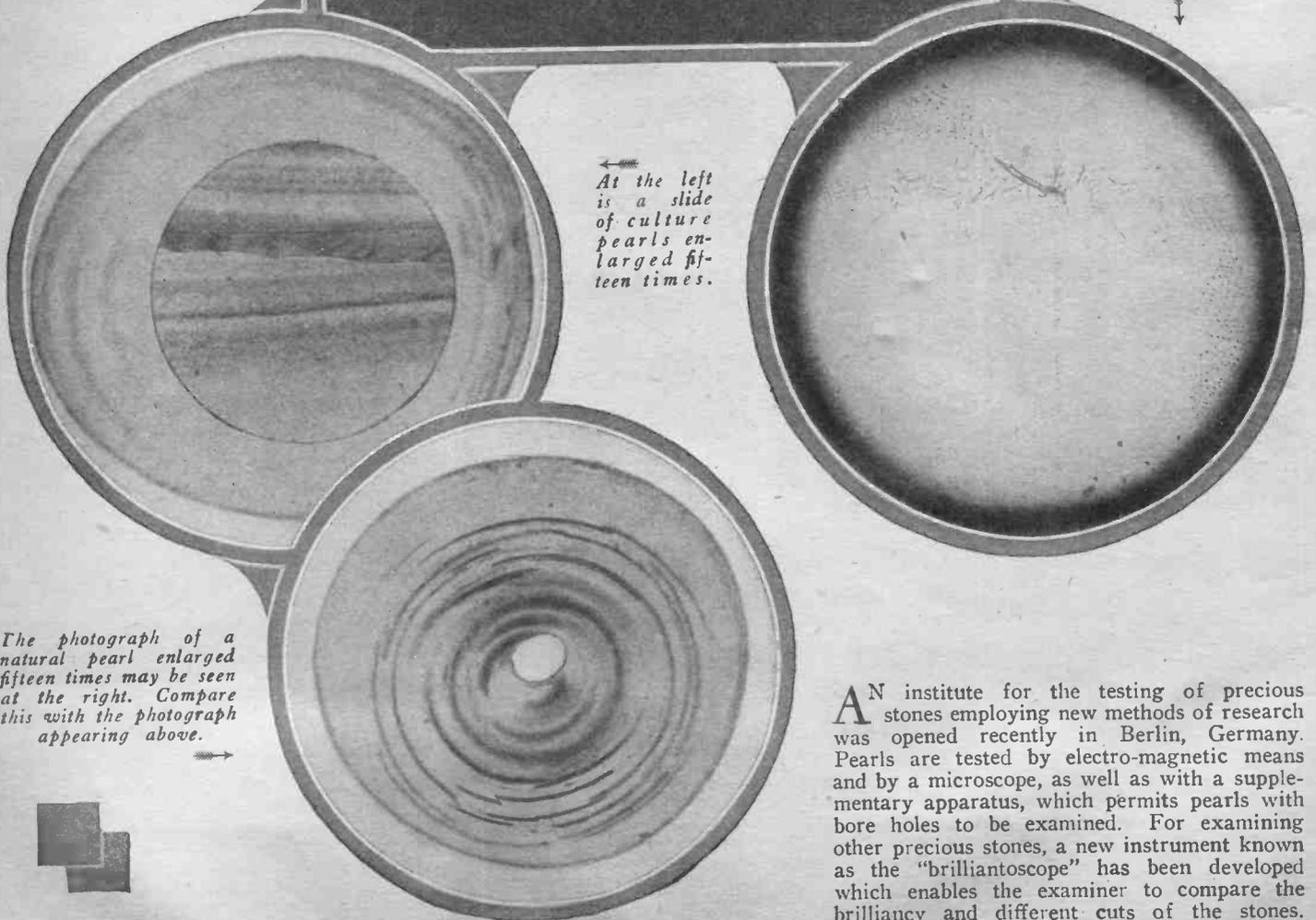
AN institute for the testing of precious stones employing new methods of research was opened recently in Berlin, Germany. Pearls are tested by electro-magnetic means and by a microscope, as well as with a supplementary apparatus, which permits pearls with bore holes to be examined. For examining other precious stones, a new instrument known as the "brilliantoscope" has been developed which enables the examiner to compare the brilliancy and different cuts of the stones.
