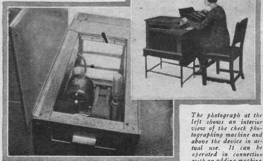
The photograph at the left shows an interior view of the check photographing machine and above the device in actual use. It can be operated in connection with an adding machine.
