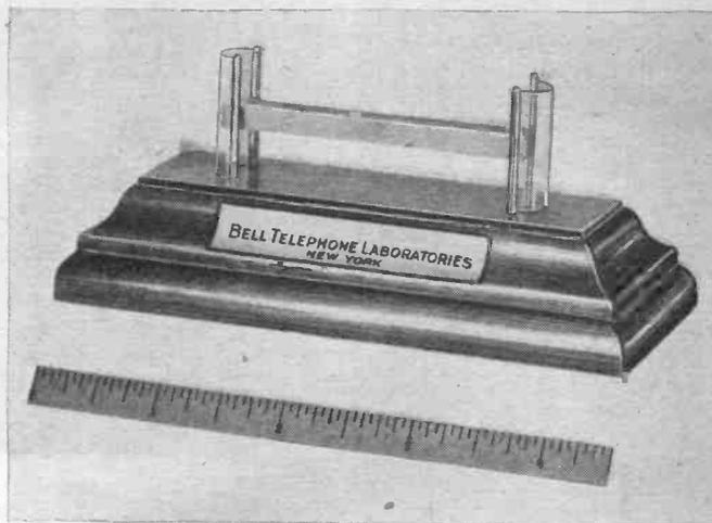
The above photograph shows the cobalt steel magnet suspended in air as if by magic. The bar is highly magnetized and is repelled by a similar bar embedded in the wooden base. Guiding channels at each end hold the levitated bar in place.
