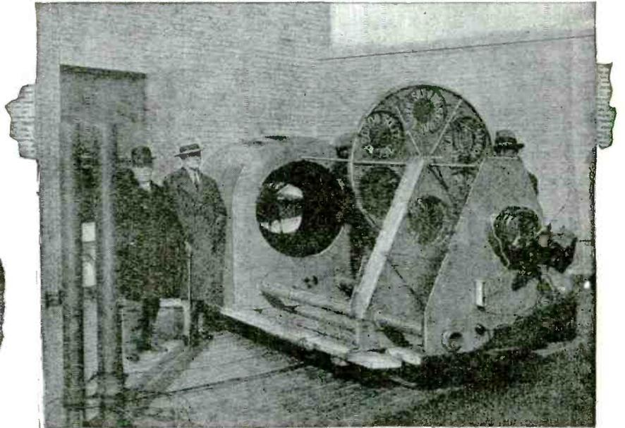
A sky advertising projectograph, a German invention recently demonstrated here, is shown in the above photo. The stencils containing the advertisements are mounted on a rotatable disc. A carbon arc light is used to project the ads on the clouds at night. Due to the rotating disc, the pictures are projected over a wide area when using the clouds as a screen.
