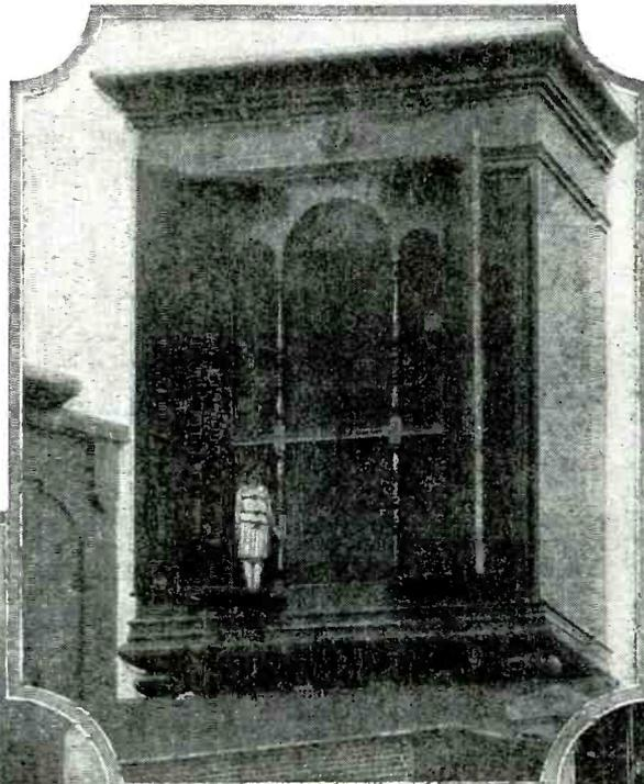
it is possible to reproduce sound with extraordinary faithfulness at a great distance. The instrument is operated by remote control, which is placed below the machine in the building upon which it has been erected. It is practically impossible for one to remain inside the cabinet.
