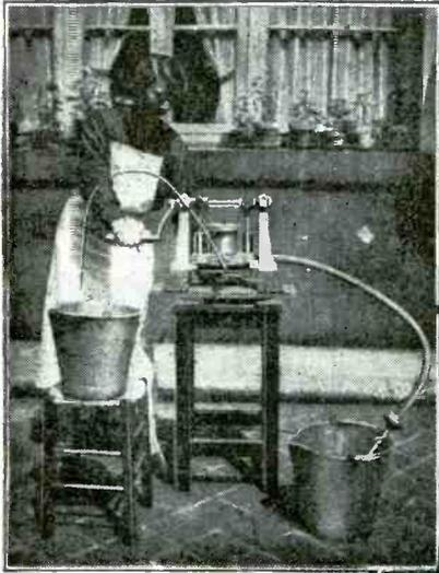
At the left is a photo of a new churn which has two double-stroke pistons connected to the main chamber in which the milk is churned. It is operated either by a lever or a handle attached to a crankshaft for alternate movement. The churn is the invention of M. Kerpinski of Paris.
