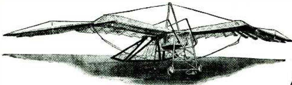
The photograph at the left shows a new wing-flapping machine or ornithopter which is propelled by foot power. The ornithopter weighs only 100 pounds and has a wing spread of 25 feet. The fuselage measures 8 feet in length. Below is George R. White, the inventor.
