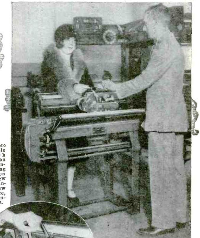
By means of the new printing machine shown above and also at the left, railroads can now print tickets for passengers when they call for them, instead of preprinting and keeping on hand thousands of tickets. The machine works like a typewriter and not only prints the ticket, but also keeps a record. The machine is shown above and at left.
