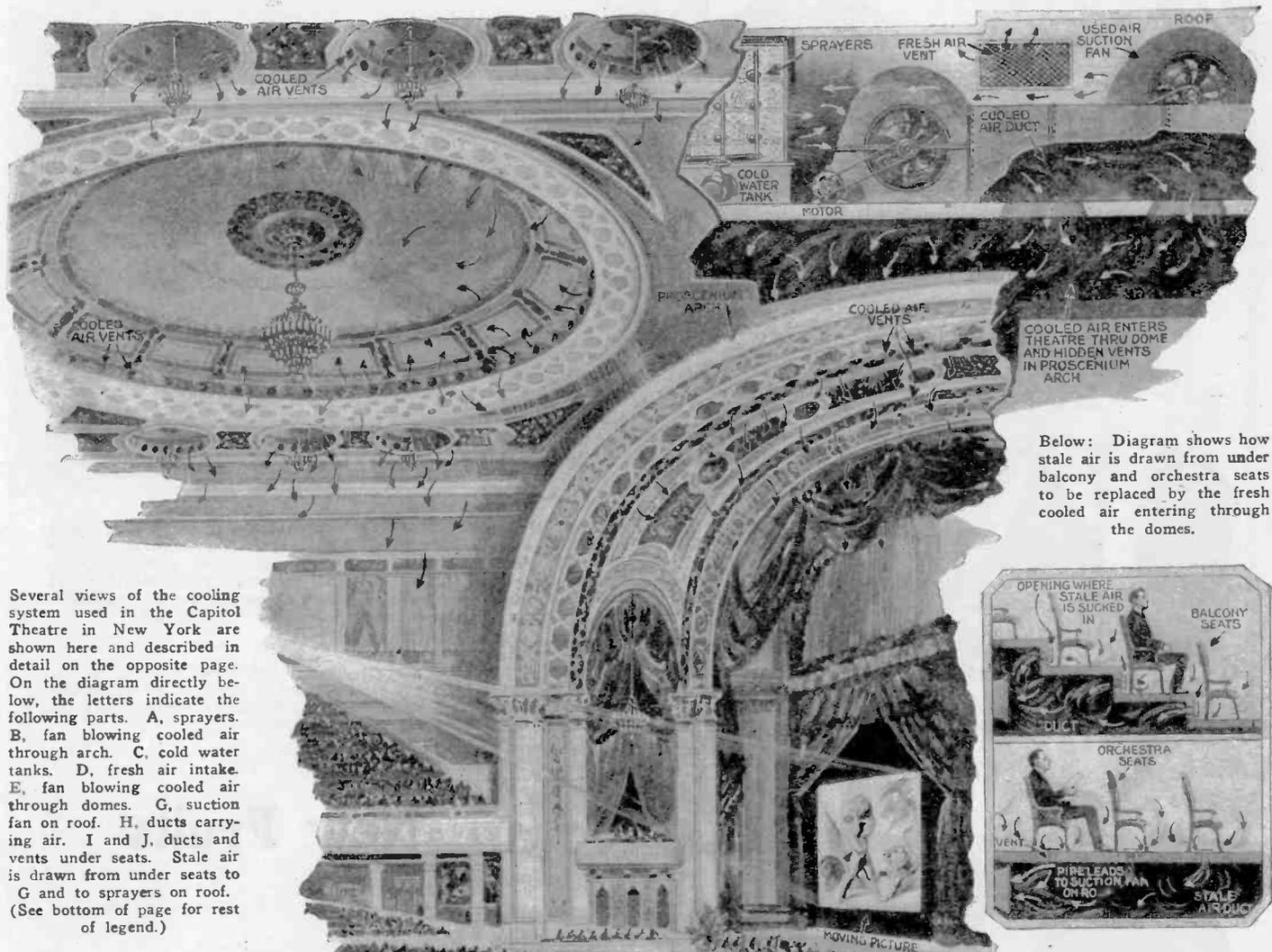
Below: Diagram shows how stale air is drawn from under balcony and orchestra seats to be replaced by the fresh cooled air entering through the domes.
