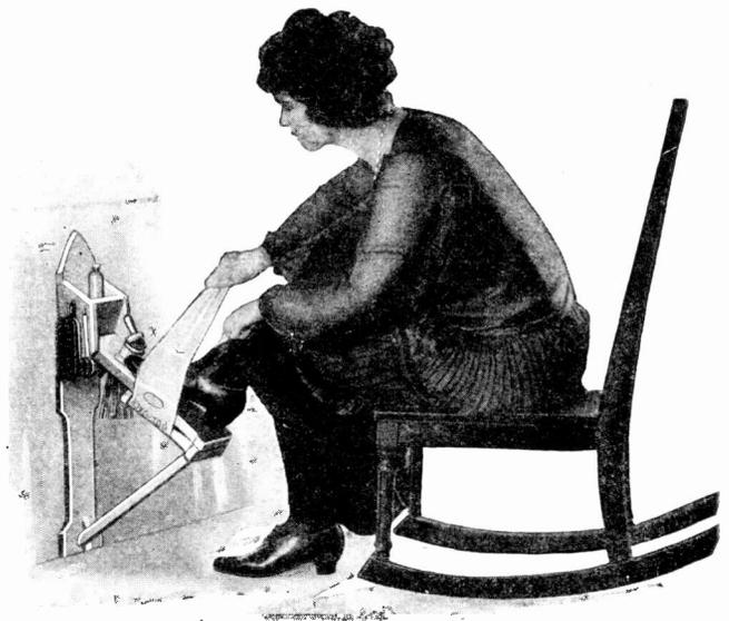
A shoe polishing device that folds up against the wall when not in use is illustrated above. When in use, the footrest can be locked rigidly at either of two heights. Under the footrest are two rollers upon which the polishing cloth moves back and forth, thus imparting a brilliant shine to the shoes. Space is provided for the polishing cloth and such accessories as cleaning liquid and paste.
