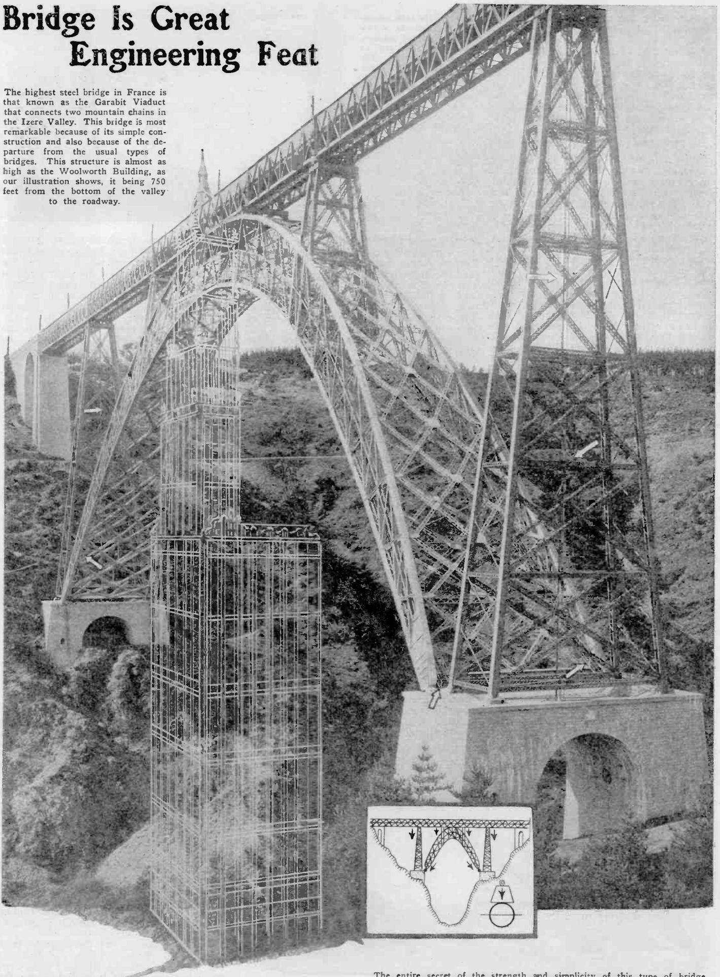
The arrows in the illustration above indicate stairways and ladders that make every part of the framework of this remarkable bridge easily accessible for inspection, painting and repairing. The entire span rests on four concrete abutments.
