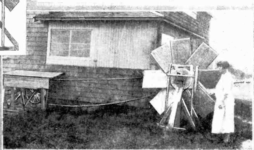
↑ An ingenious mechanic of Brewster, Mass., has succeeded in harnessing wind power to pump water for his country home. He made up a very simple wind mill that is shown in the photograph and drawing above, and hitched to the mechanism of a bicycle by means of a belt. The crank of the latter actuates a pump and it is said that 20 minutes' work by this device will pump enough water to last for two weeks. In a high wind, a buzz saw can be operated by the wind mill.
