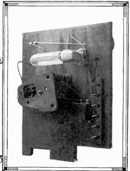
In the photo to the left is shown a part of the phonograph cabinet housing battery connections and amplifying transformers for operating the loud speaking apparatus. A switch is provided to control the amount of amplification to be obtained.
