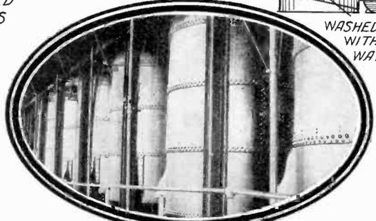
Photo at the right shows a large digester installation. Sometimes an individual digester is sufficiently large to hold thirty cords of wood. Digestion forms a part of the acid process used in the manufacture of sulphite pulp.
