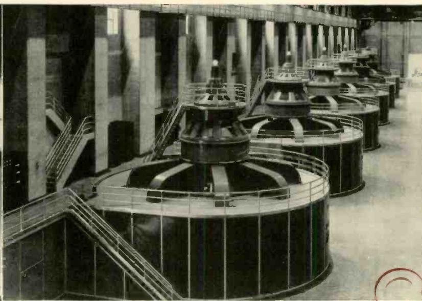
Installation of the 82 500-kva units (above) at Hoover Dam began in 1933. In each wing at Grand Coulee (left) will be nine, 108 000-kva, 120-rpm units all installed or under construction.
