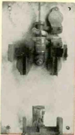
Left, one of the earliest circuit breakers on a marble base. Below, breaker built for original Niagara Falls system.
