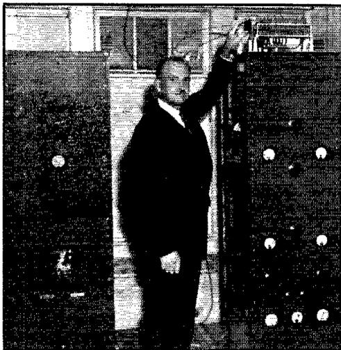
Frank Carter, W2AZ, of East Rockaway, Long Island, N. Y., is the first to break into the DXCC with all stations worked on 'phone. A vertical collinear two half-waves in phase and two 8-element horizontal stacked arrays are supported from the three 85-foot poles available. The receivers are Super-Pro and HRO with an acorn-tube preselector. The transmitter winds up with a pair of 300T's, modulated by a pair of 250TH's, with 2100 volts on the plates.
