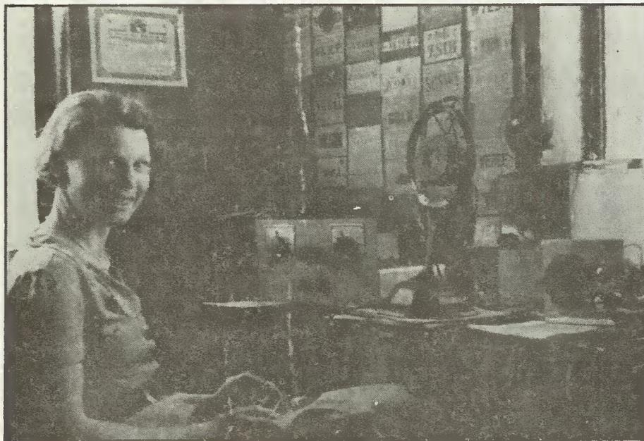
Eileen Heightman, with the home built 10 metre receiver and associated equipment, operating G6DH, one of the earliest amateur radio stations to explore the 10 metre band.
