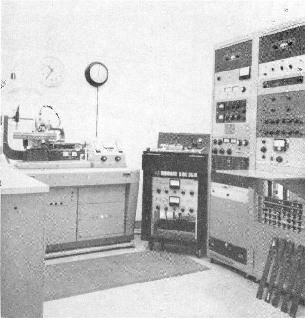
Figure 3. A view at Century Recording where the engineer stands in the cutting room. The sound-level meter was placed at ear level in front of the cutting lathe.
