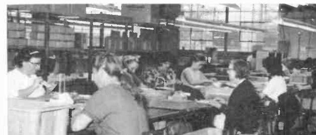
Figure 9. The loaded cassettes are checked before they are fed to a machine that will seal the cover to the body. Then other automated equipment labels the cassette, places it in a case, and wraps it.
