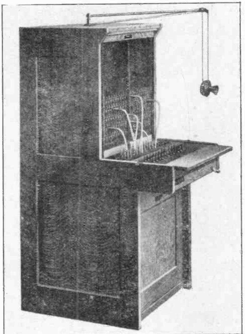
Fig. 17. Side view of a magneto type switchboard with some of the plugs in place in the various line jacks.
