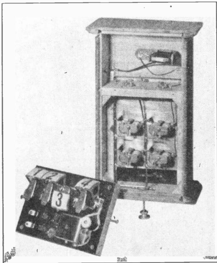
Fig. 4. Photograph showing the inside parts and construction of two common types of annunciators.
