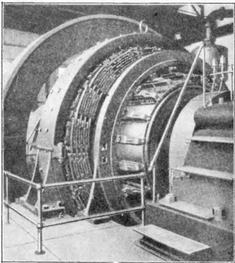
Fig. 5. Large D. C. generator. It is rated as follows, 2000 Kw., 250 V., 8000 l. After carefully reading the pages on units and symbols, you should easily understand this rating.
