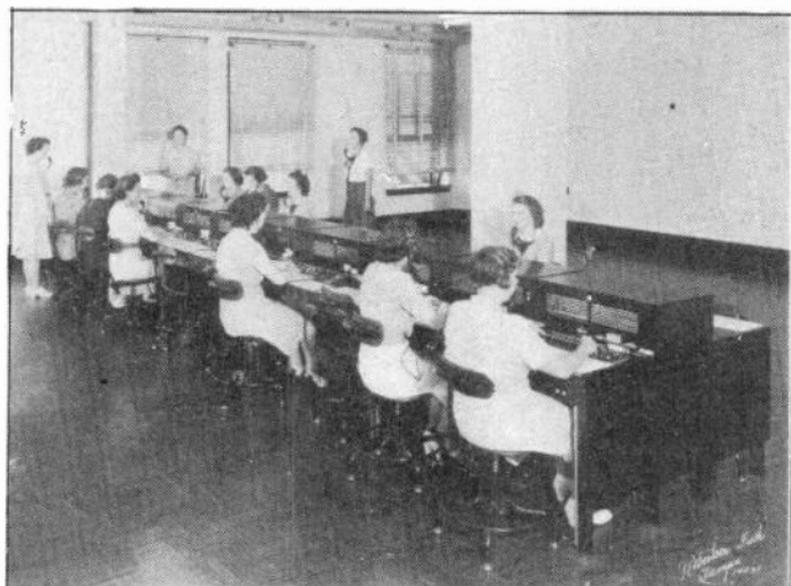
Fig. 22. This photograph shows a section of a large manual telephone exchange. Each operator controls a section of the board
