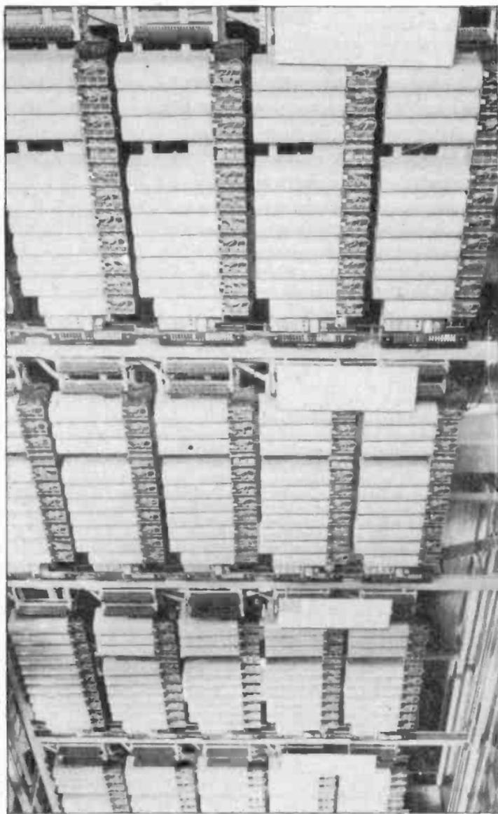
Photo shows Strowger (Step-By-Step) Dial Telephone Switching Equipment. Note the compact neat arrangement of all parts and equipment. (Photo Automatic Electric Co.)
