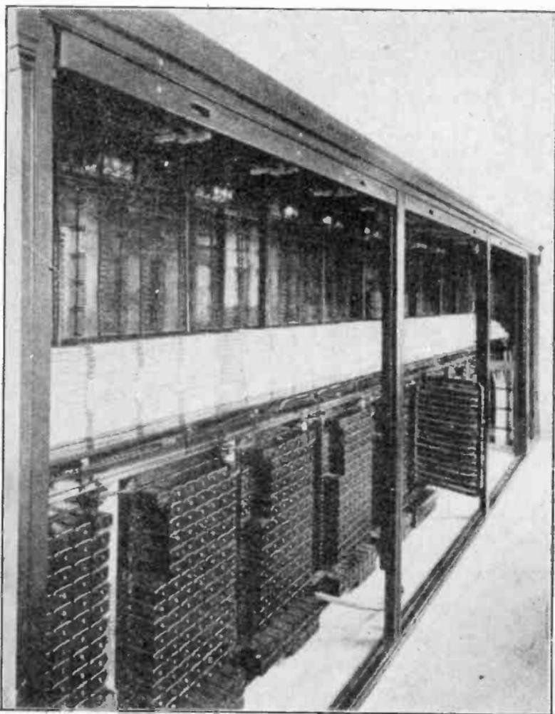
**Fig. 23.** Rear view of a central exchange switchboard. Note the very neat and compact manner in which all parts and wires are arranged to simplify connections and testing of such exchange units.
