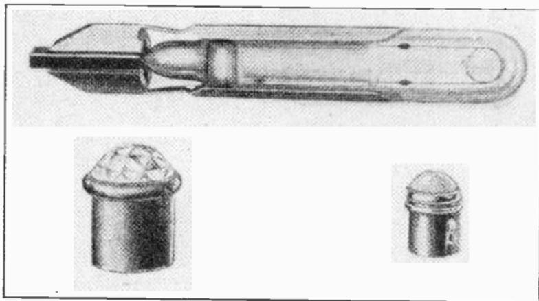
Fig. 11. The upper view shows one of the special telephone switchboard lamps, and below are shown two types of glass caps, or bull's-eyes used with such lamps.
