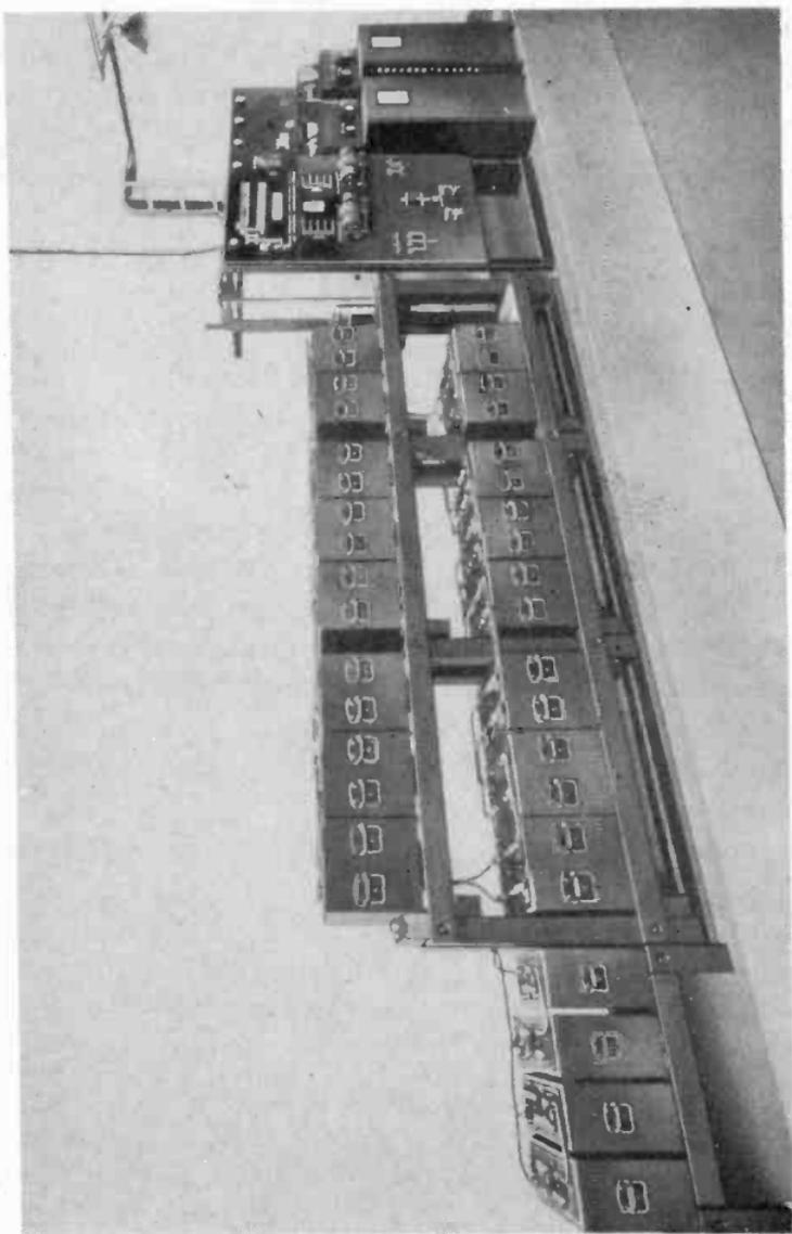
**Fig. 53. Storage Batteries Which Furnish Electric Power for a Telephone System.**
