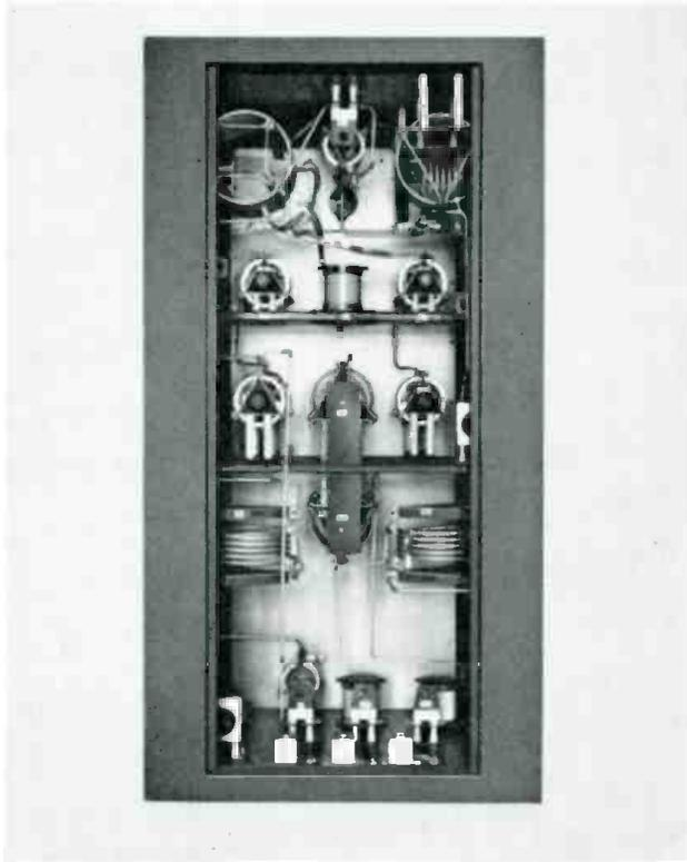
Phasing Cabinet showing simplicity of design and layout. Custom equipment provides maximum stability for dependable AM operation, for three tower, 10-KW stations.
