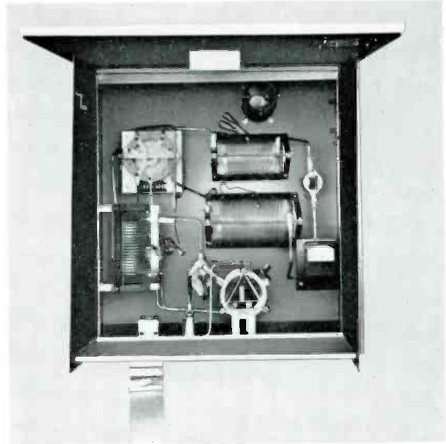
Line Terminating Unit installed in weatherproof cabinet.
