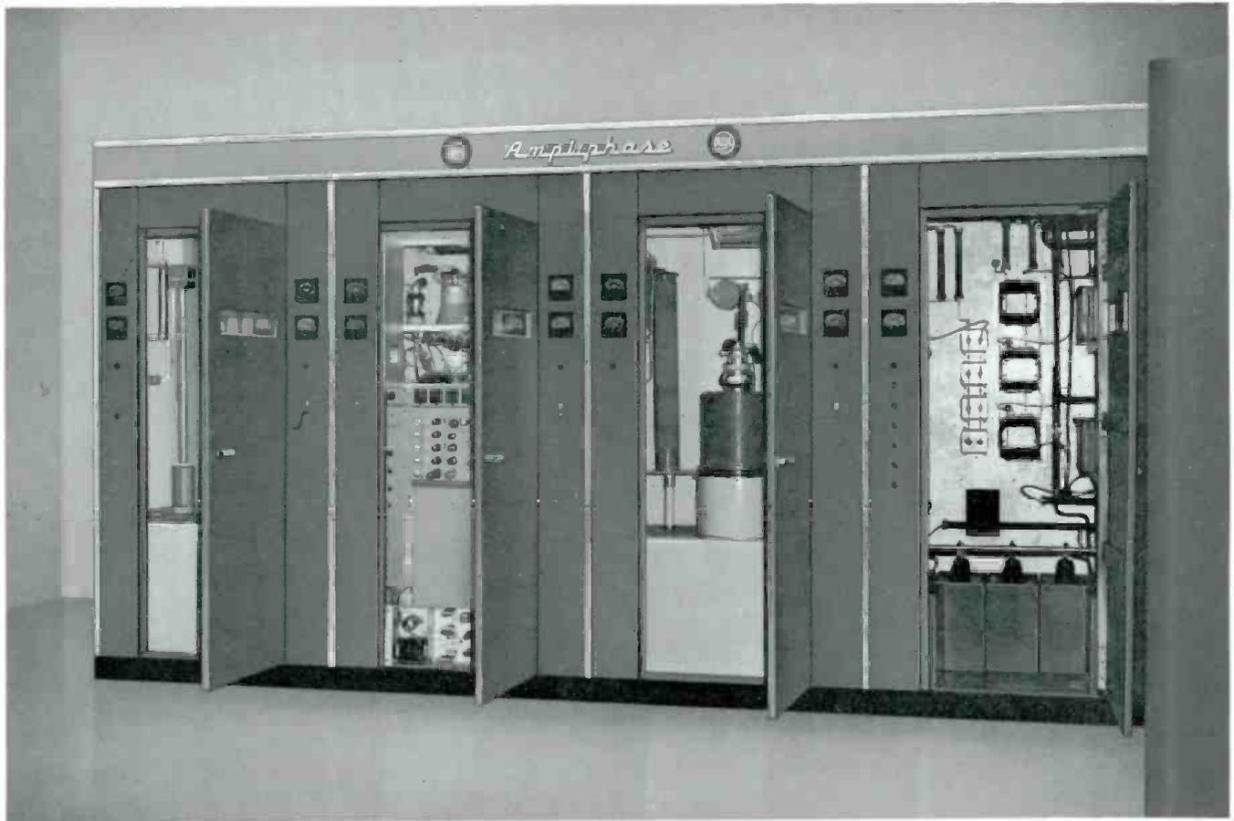
Compact in-line construction of BTA-50H showing left to right, first power amplifier, exciter, second power amplifier, and rectifier-control cubicles with doors open.
