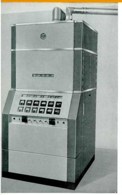
One of the power amplifiers of the TT-100AH showing front panel with tuning motor switches, individual tube meters, tuning indicators, switches and status lamps. Tubes, located behind hinged access doors, are of plug-in type for rapid change.
