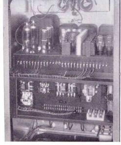
Sectional Rear View Showing Center Chassis and Relay Chassis
