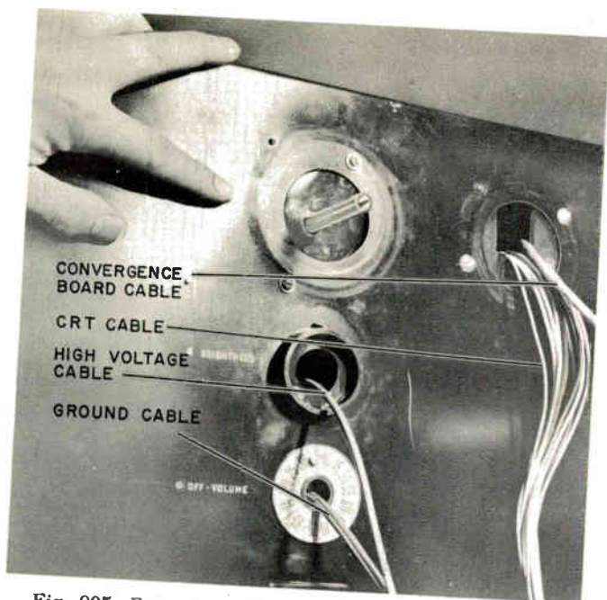
Fig. 905. Extension cables protrude from control holes in mockup set. Bushings and dial plates from junkbox keep insulation from chafing on edges of holes. Plastic insert nearest hand is convenient for holding cables when mockup is not used.
