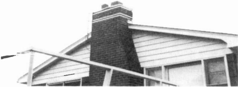
Fig. 13-6. JFD and RCA antennas mounted on the author's chimney, one above another. The upper antenna (RCA) supplies two outlets, while the larger (JFD) delivers good signals to four. No power is used, and 11 Washington-Baltimore stations are received, most of them very well.
