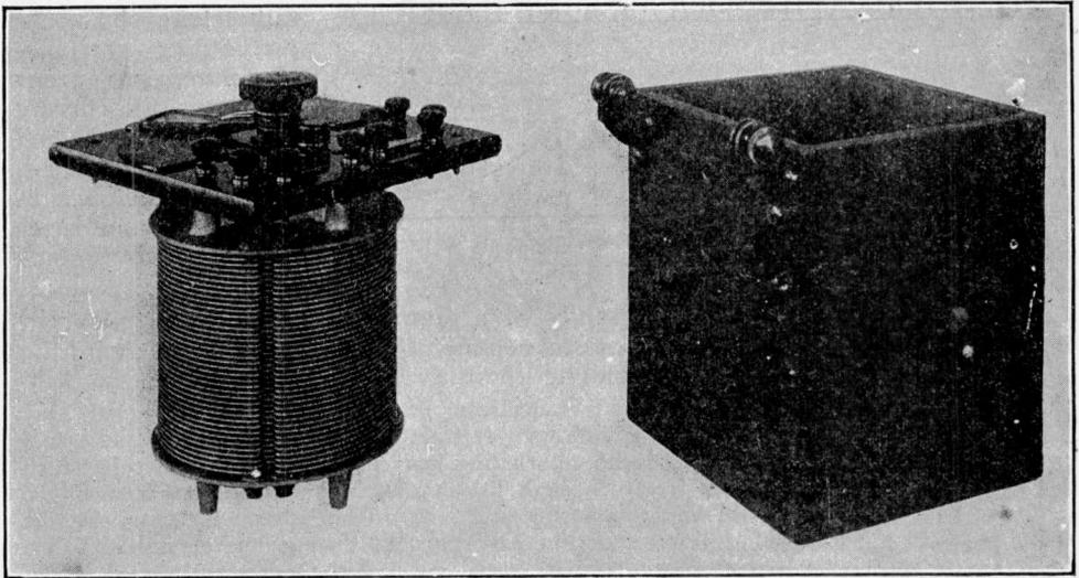
Fig. 147a—Variable Condenser for Receiver Circuits.
