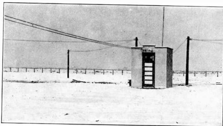
FIG. 46.—Transmission-line antenna coupling. Radio-frequency power is carried over a long transmission feed-line from the transmitter to the main antenna system when the latter is located several hundred feet or more from the transmitter building. This system provides an effective suppressor of existing harmonics. The antenna coupling and tuning equipment required to couple the transmission line to the antenna system is housed in the small shed.
