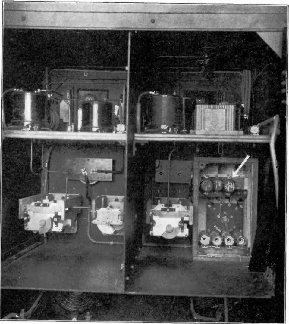
FIG. 29.—A view of the quartz crystals installed at WEA F to maintain stabilized frequency. Three crystals are shown above, as indicated by the white arrow, although only one is used at a time—the remaining two being held for emergency.
