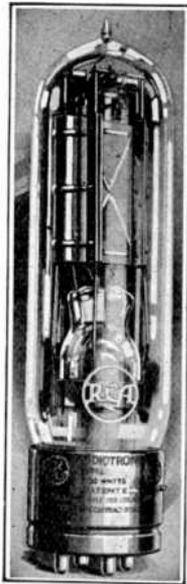
FIG. 48.—A 50-watt transmitting tube.
